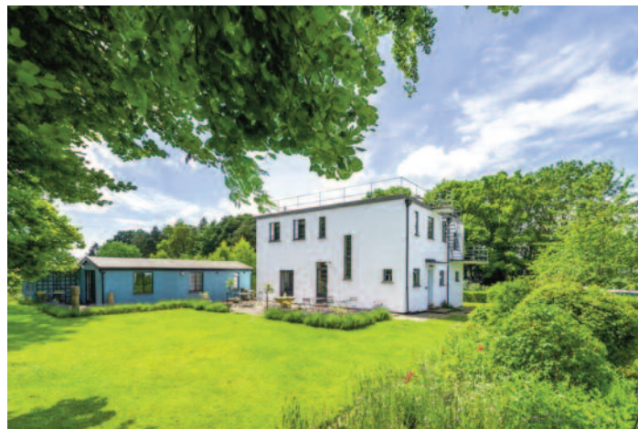
The former control tower at RAF North Creake
